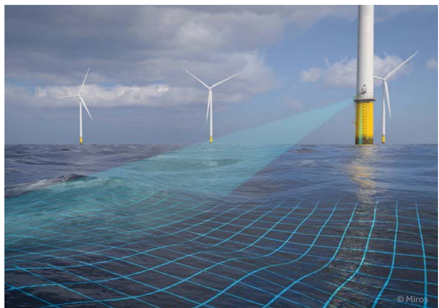
Continuous monitoring of dynamic forces, such as waves, on turbines is essential to ensuring the longevity of these massive structures. In turn, this guarantees that developers can maximize the return on their substantial investments
